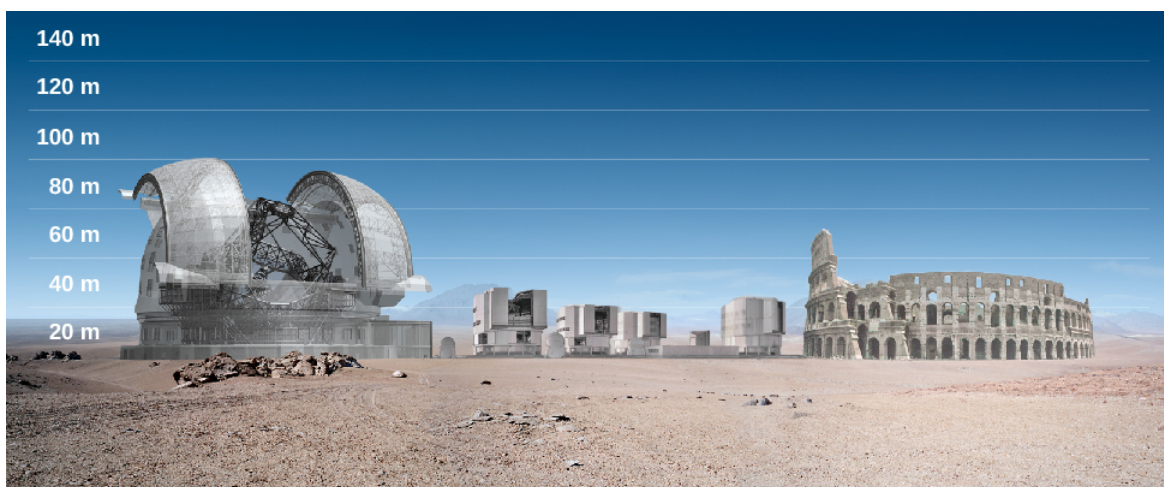
Figure 29.1.5 European Extremely Large Telescope, European Very Large Telescope, and the Colosseum. The European Extremely Large Telescope (E-ELT) is currently under construction in Chile. This image compares the size of the E-ELT (left) with the four 8-meter telescopes of the European Very Large Telescope (center) and with the Colosseum in Rome (right). The mirror of the E-ELT will be 39 meters in diameter. Astronomers are building a new generation of giant telescopes in order to observe very distant galaxies and understand what they were like when they were newly formed and the universe was young.
