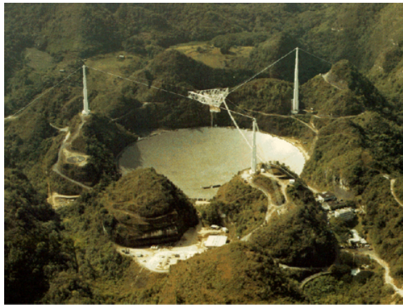
Figure 6.4.6 Largest Radio and Radar Dish. The Arecibo Observatory, with its 1000-foot radio dish-filling valley in Puerto Rico, is part of the National Astronomy and Ionosphere Center, operated by SRI International, USRA, and UMET under a cooperative agreement with the National Science Foundation. (credit: National Astronomy and Ionosphere Center, Cornell U., NSF)
