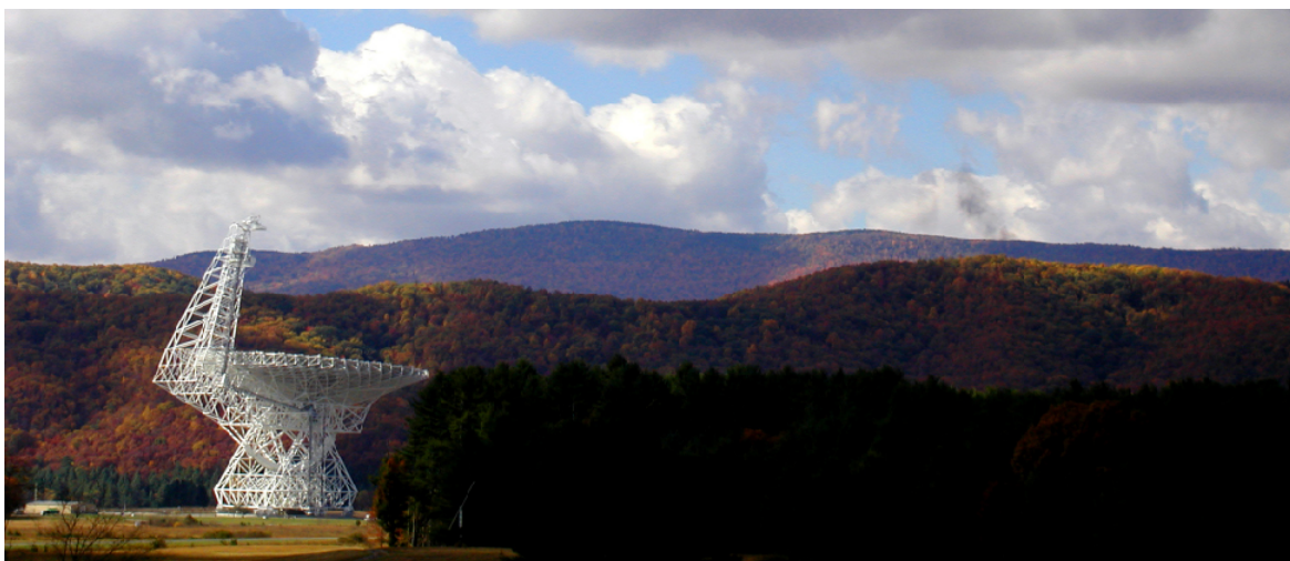
Figure 6.4.3 Robert C. Byrd Green Bank Telescope. This fully steerable radio telescope in West Virginia went into operation in August 2000. Its dish is about 100 meters across. (credit: modification of work by “b3nscott”/Flickr)
