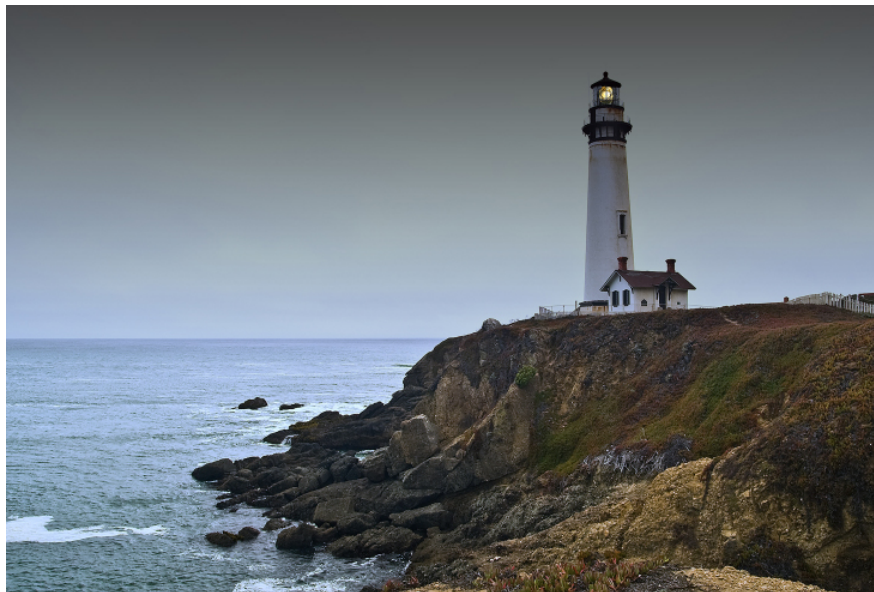
Figure 23.4.2 Lighthouse. A lighthouse in California warns ships on the ocean not to approach too close to the dangerous shoreline. The lighted section at the top rotates so that its beam can cover all directions. (credit: Anita Ritenour)
